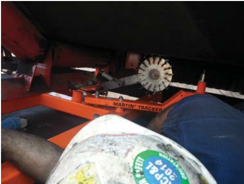
MartinPLUS® Installation Crew installing the Martin® Tracker™ Reversing.
