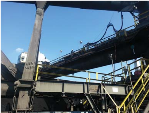
Mid American Energy 's reclaim belt was mistracking during the reclaim and coal stack out process.
