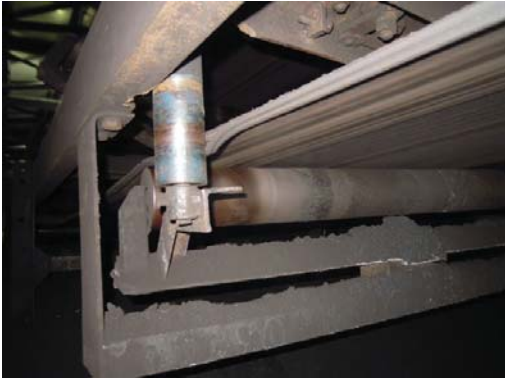
The Luling mine was experiencing belt misalignment on one of their conveyors resulting in heavy damage to the belt edge.
