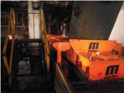
MartinPLUS® Technicians installed transfer point solutions to address the problems.
