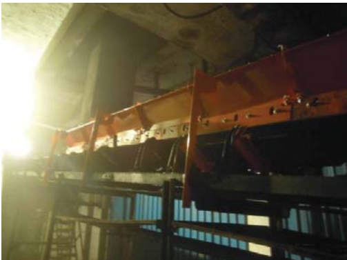
Since the installation was completed, visible dust within the facility has been drastically reduced.
