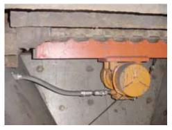
To improve coal feeding, a new vibrator and channel mount were installed on a vibrating feeder pan at F. B. Culley Station.
